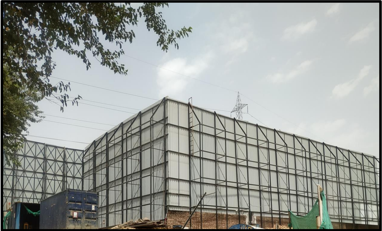
Front - Inside Barricading
